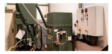
The blast room took two weeks to install and commission. With Hodge Clemco's installation team onsite to deal with any issues or queries regarding the build. The blast room is acoustic, so dampens the noise in the rest of the factory when workers are blasting. The blastroom is fiitted with an external dust and recovery system.
